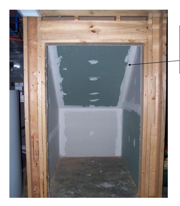
Drywall required on the underside of basement stairs when a closet/storage is being added.
