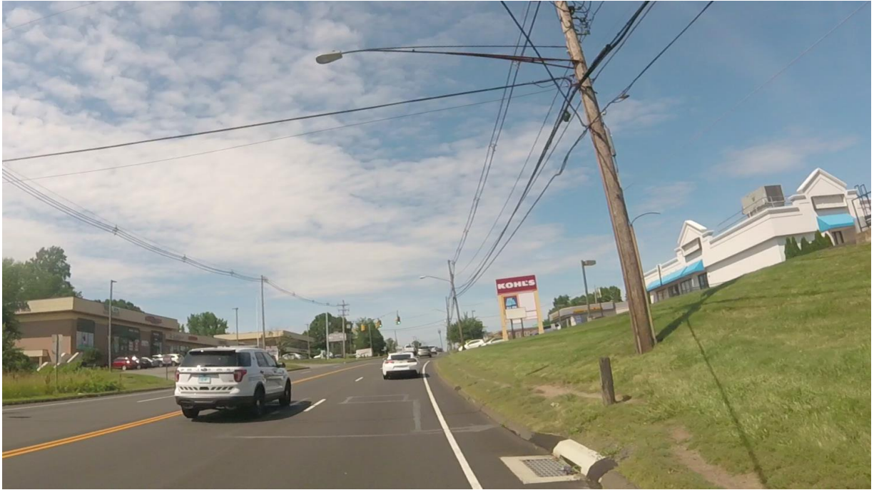
#31 Northbound Route 5, At State Road 150
