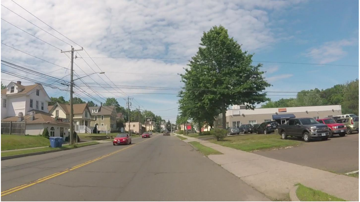
#23. Northbound Route 5, Between Ann St. and Hall Ave.
