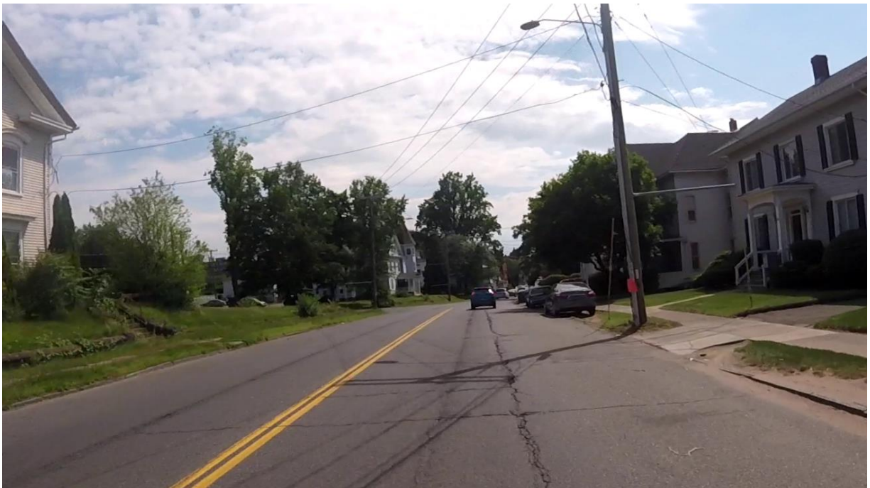
#16 Southbound Route 5, Between Dayton St. and Wall St.
