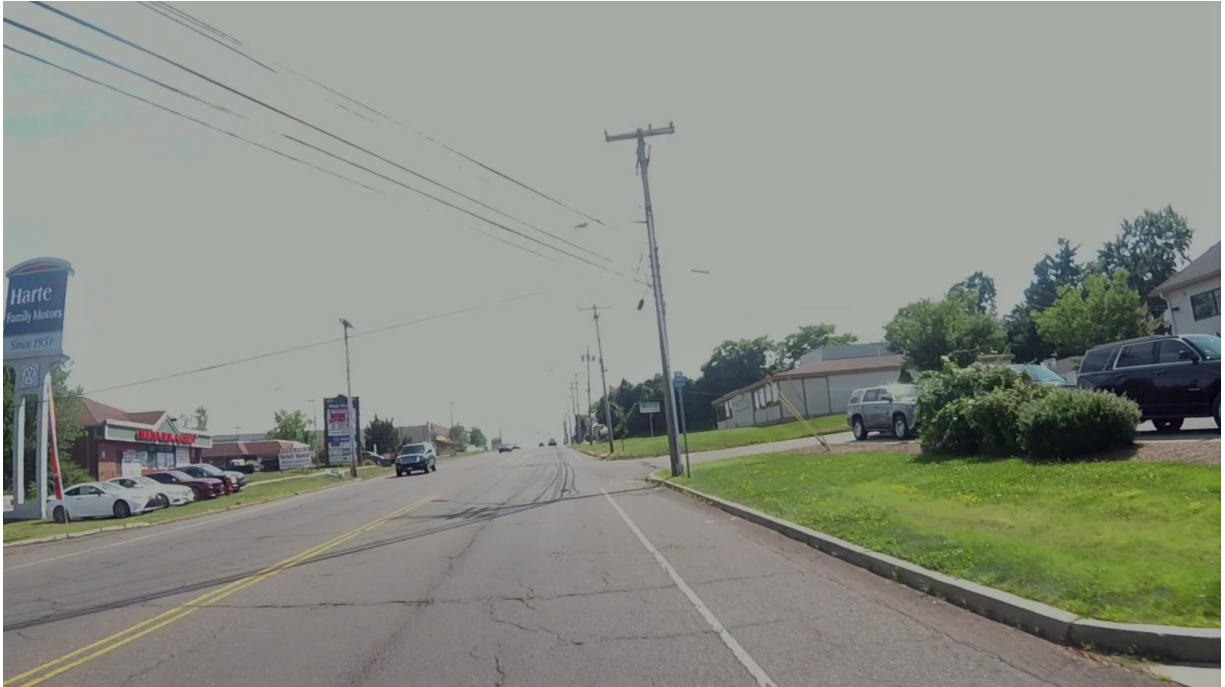
#29 Southbound Route 5, Between Gypsy Ln and North Dr. to TLP
