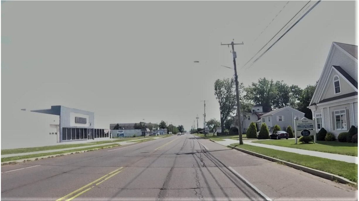
#27. Southbound Route 5, Between Hall Ave. and Gypsy Ln
