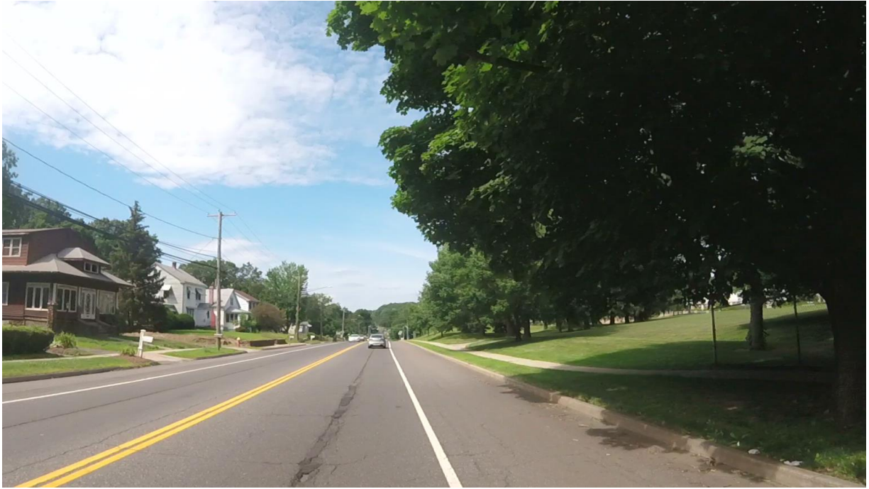
#3 Northbound Route 5, North of Robin Hill Road
