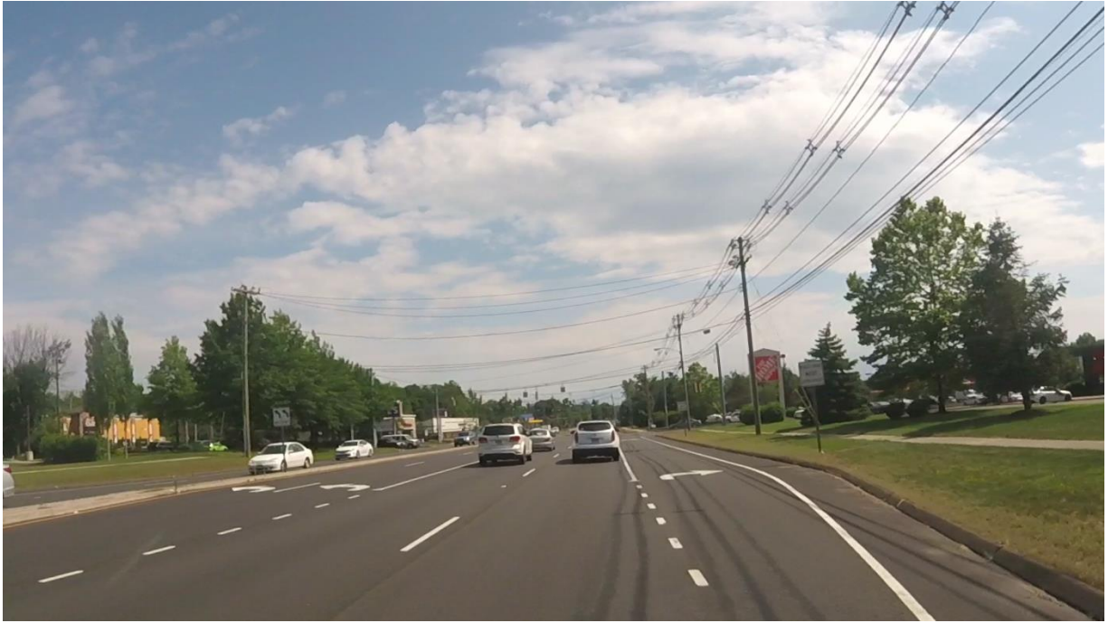
#33 Southbound Route 5, Between Circle Drive and Neal Road
