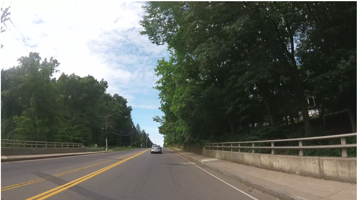
#6 Northbound Route 5, Between Blackstone and Britannia St (2)
