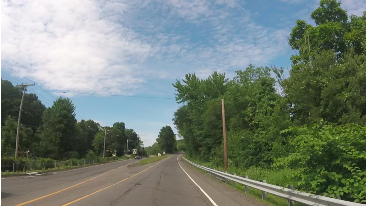
#1 Northbound Route 5, North of Stoneycrest Drive
