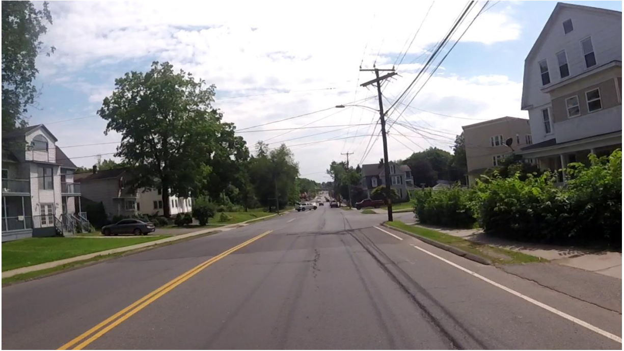
#7 Southbound Route 5, North of Sherman Avenue
