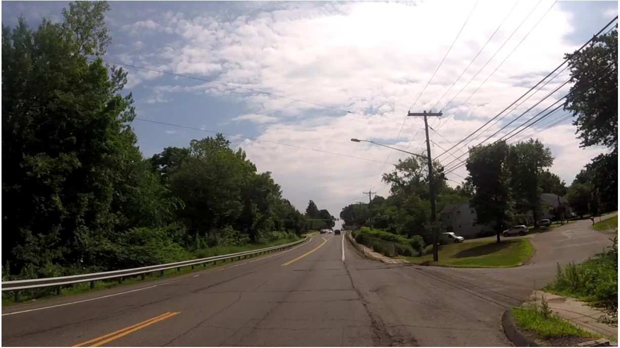
#1 Southbound Route 5, North of Stoneycrest Drive
