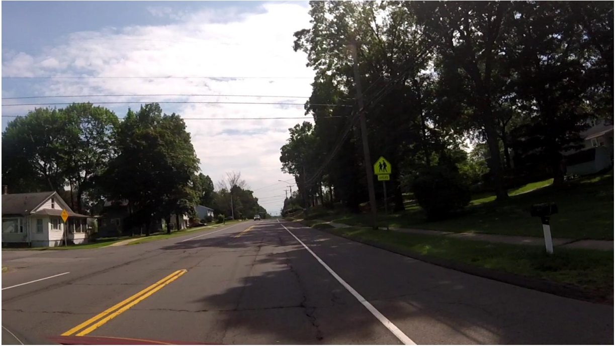
#3 Southbound Route 5, North of Robin Hill Road
