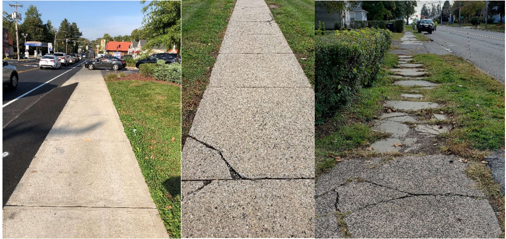
Examples of sidewalks in good, fair, and poor condition along the Route 5 corridor.
