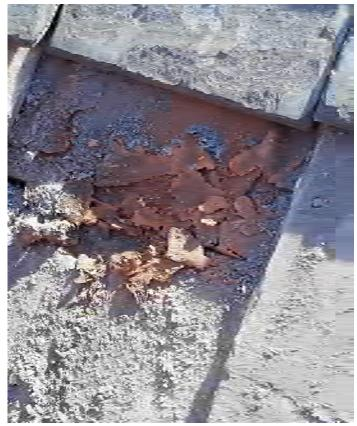
West Roof: Vapor Barrier Under Slate Shingle
