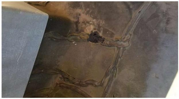
East Lower Roof (2<sup>nd</sup> Floor): Presumed PCBs Tar sealant on rubber
