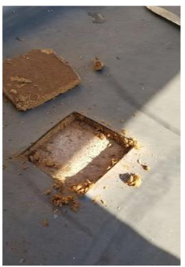
East Lower Roof (2<sup>nd</sup> Floor): rubber layer on wood core on concrete
