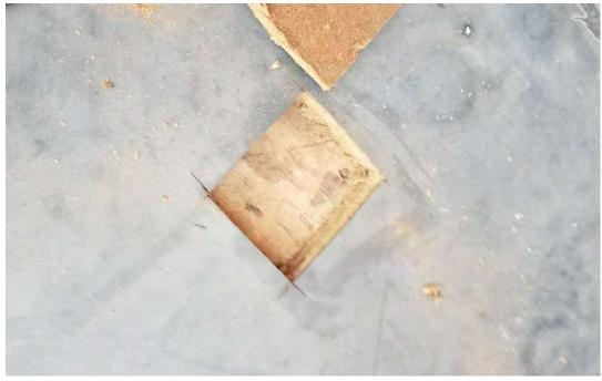
South Lower Roof ( $2^{nd}$  Floor): Rubber on wood boards layered to make slope for water runoff.
