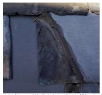
North Roof: Presumed PCBs Black Caulk on Slate Roof Shingle (Repair)
