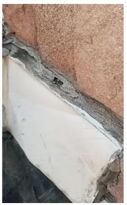
West Lower Roof (2<sup>nd</sup> Floor): Presumed PCBs Brown Caulk on metal/copper
