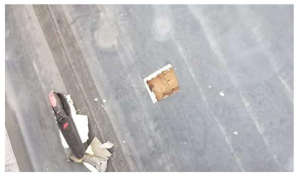
Center Roof: Rubber on Styrofoam Insulation.
