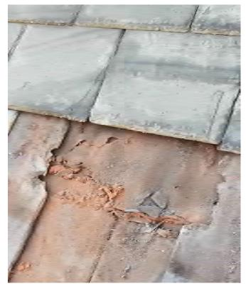
North Roof: Vapor Barrier under Slate Shingles.
