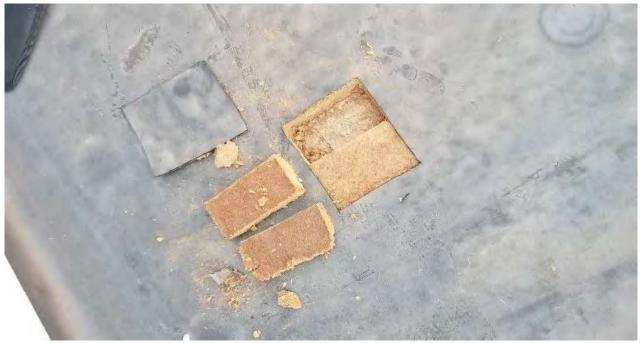
West Lower Roof (2<sup>nd</sup> Floor): Rubber on wood core on cement.
