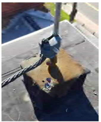
Center Roof: Presumed PCBs Grey Sealant on Lighting Rod
