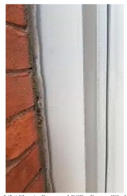
South Lower Roof (2nd Floor): Presumed PCBs Brown Window Frame Sealant
