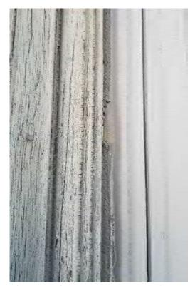
West Lower Roof (2<sup>nd</sup> Floor): **Asbestos-Containing** Brown Window Frame Sealant (Presumed PCBs)
